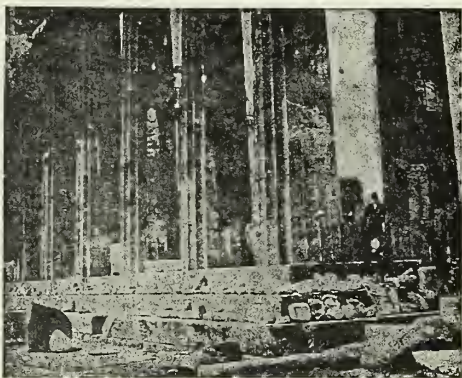
FIG. 109.—PHOTOGRAPHIC EFFECT OF CURVED STYLOBATE AND COLUMN OF THE PARTHENON.
